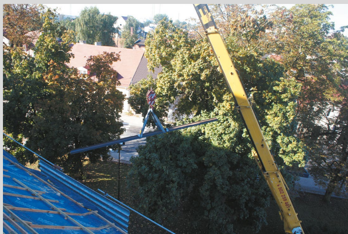
Transport belek na poddasze
